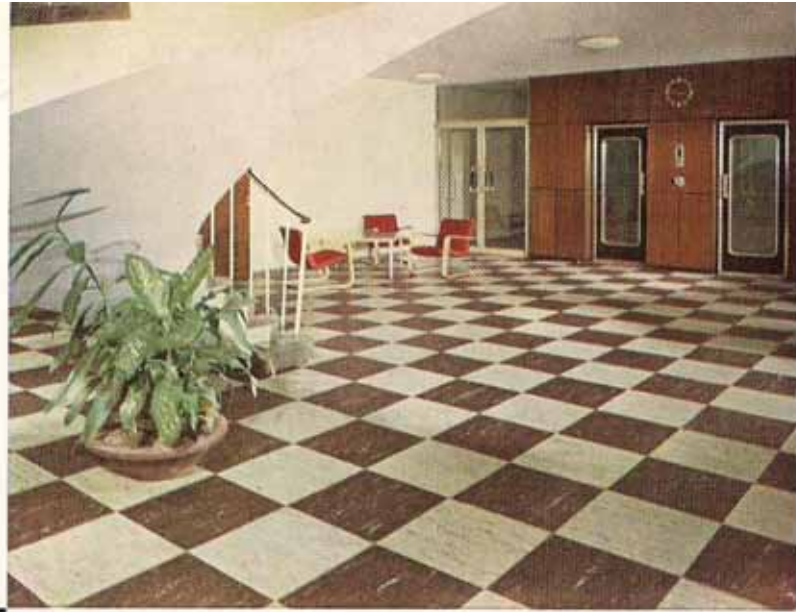
Lobby: MIPOLAM floor covering, chessboard pattern. Elevator faced with ULTRAPAS panels, macoré wood pattern
