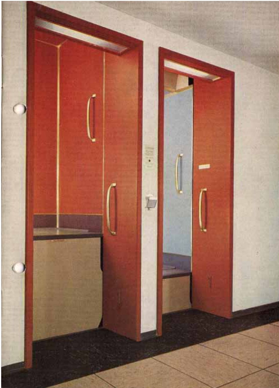
Paternoster elevator; interior lining, floor, and edging made from MIPOLAM
