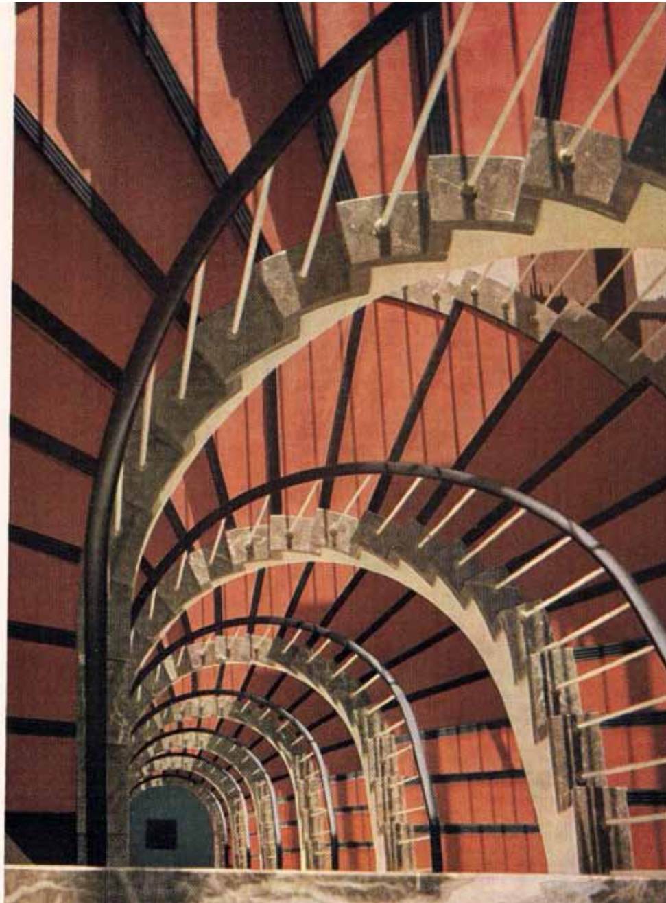
View from top of staircase: MIPOLAM treads, edges, and hand rails
